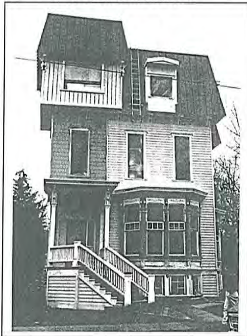
False mansard roof
