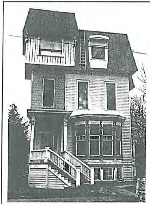
False mansard roof
